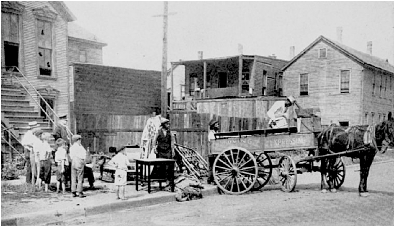
Family leaving damaged home after the Chicago race riot of 1919
